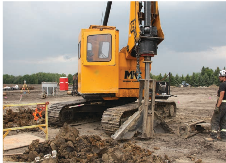
A swamper and a driller working together to safely install a belling tool
