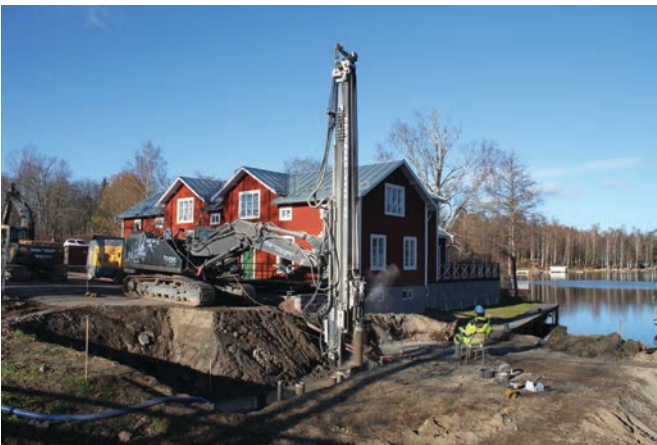
Sweden's FDS AB micropiling with a DT145 EC300
