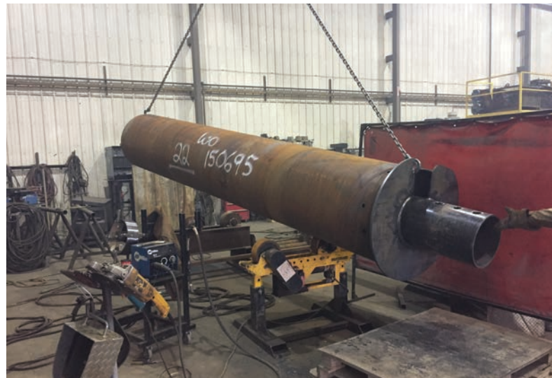
A bucket pile being manufactured
